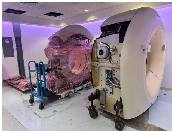
The unit had to be expertly removed in pieces, each of which could weigh around 2 tons.
